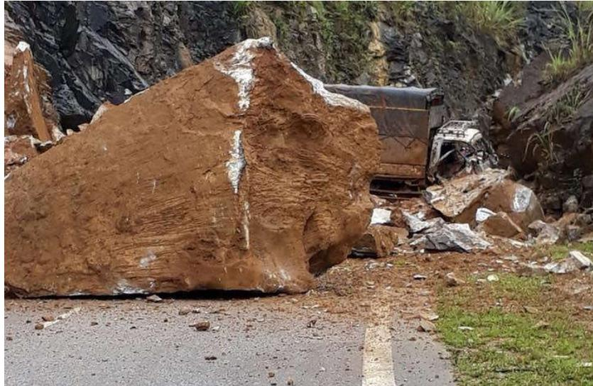
**Figure 1: Rock failure block at the km 116 + 100 on the 3B highway**
