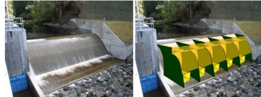
Figure 2. (Left) A human engineered Weir, (Right) A human engineered power harvesting Weir.
